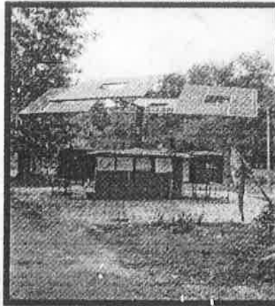
Solar Installation at Shatrunda Village, Kheda for Safe Drinking Water
